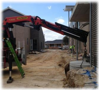
Panthers Concrete Tanks are constructed to Australian Standards AS 3735 Concrete Structures for Retaining Liquids AS 3600 Concrete Structures
